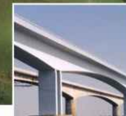
NAIGAON E/W BRIDGE
